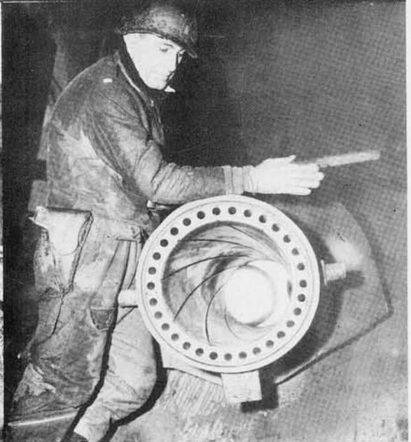
Top: General view of Sturmmörser. Above: The Raketenwerfer 61 as mounted on vehicle. Right: The projector, showing method of rifling.
