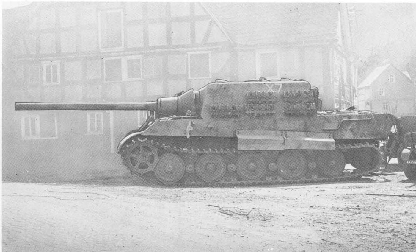
The Jägdtiger was the most formidable self-propelled anti-tank gun used by the Germans. It consists of a 12.8 cm PJK 44 (L/55) (less muzzle brake), mounted on a Tiger B chassis.
