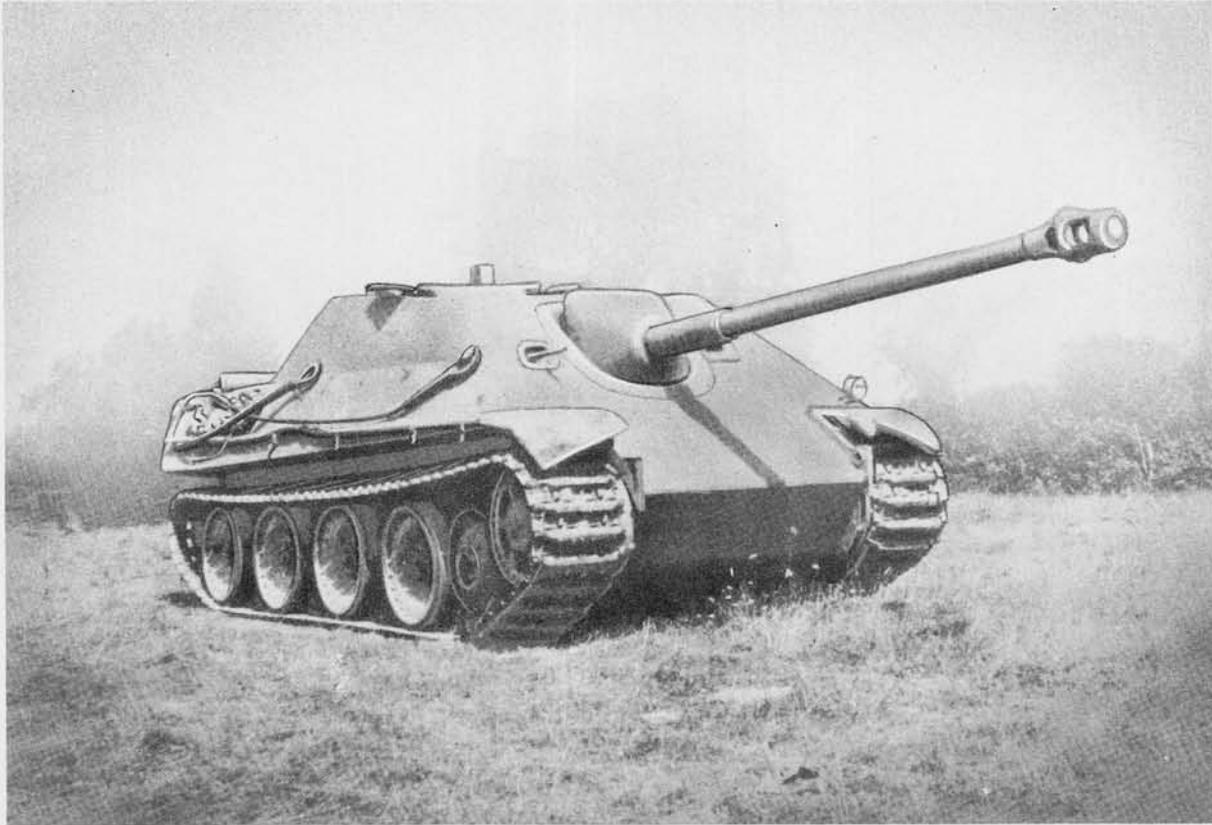
The standard Model A Panther chassis is used for building this vehicle. The vehicle embodies all of the engineering principles and methods of design accumulated by the Germans up to the time of its production, and is quite effective as an antitank or assault weapon.
