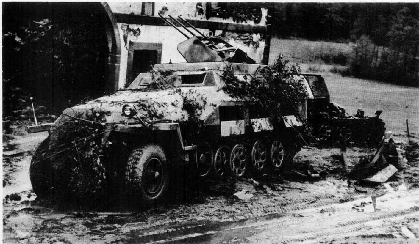
This is the 3-ton, armored semitrack mounting triple 15 mm or 20 mm heavy machine guns of the Model 151 aircraft type. The equipment is an assault weapon intended for ground combat, and engagement of low flying aircraft is a secondary role.
