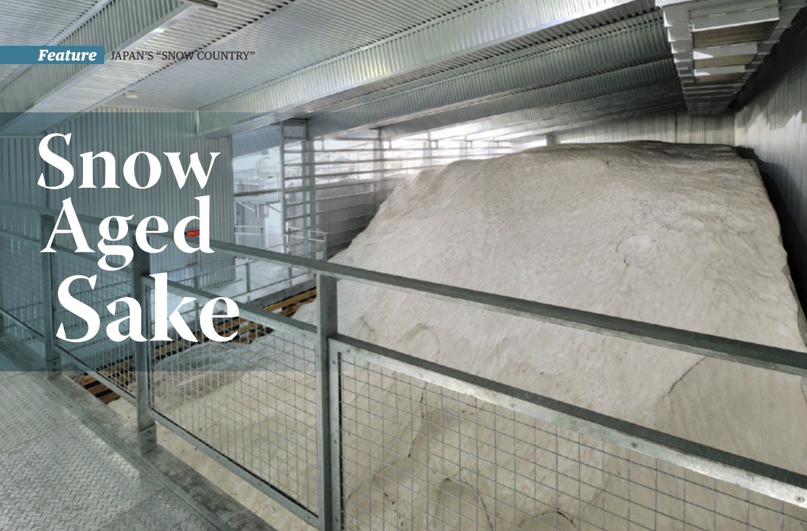
Inside the yukimuro (snow cellar), where up to 1,000 tons of snow are stored
