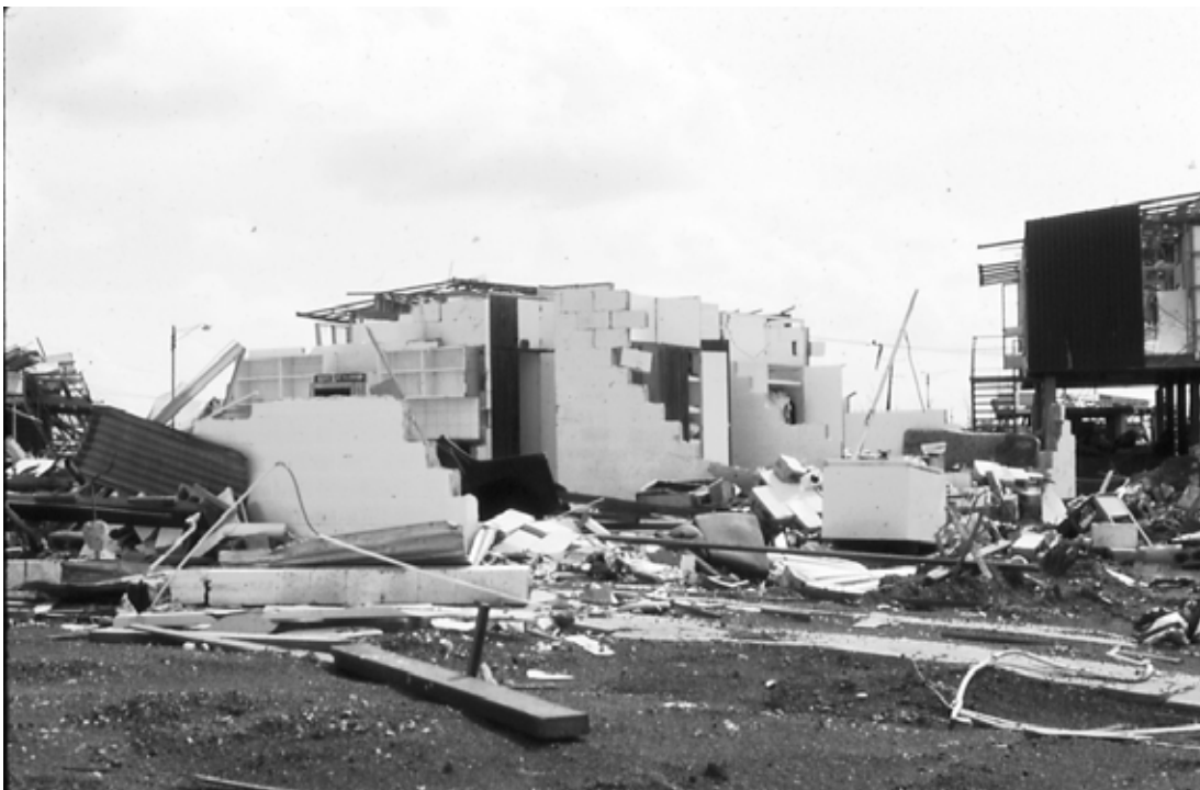
Fig 5.17 - Collapse of hollow block home
