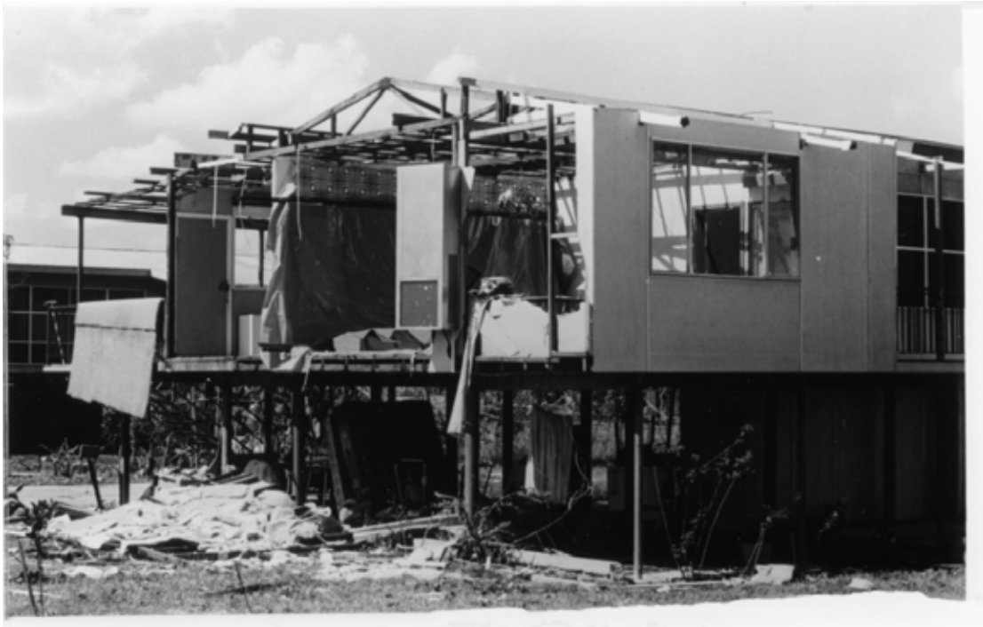
Fig. 5.7 - End wall blown out
