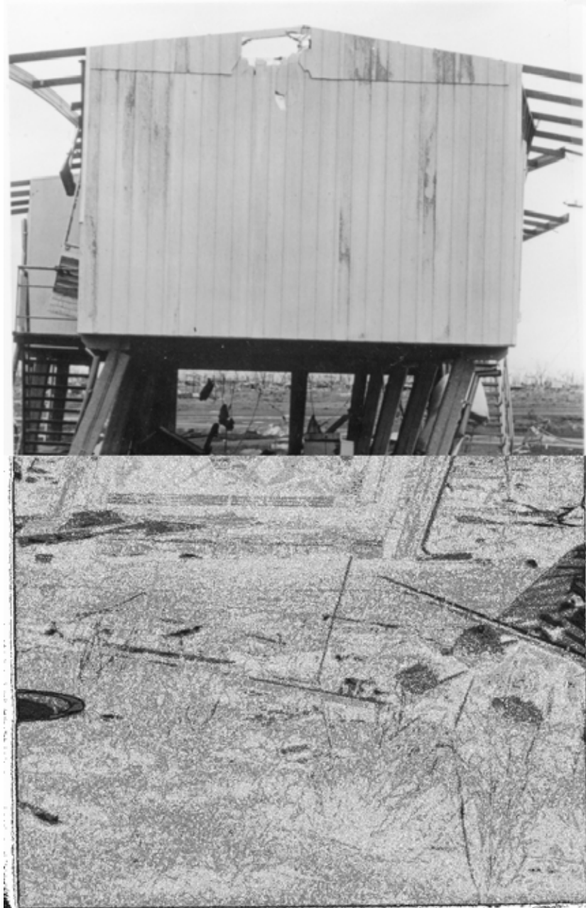
Fig. 5.11 - Failed pier
