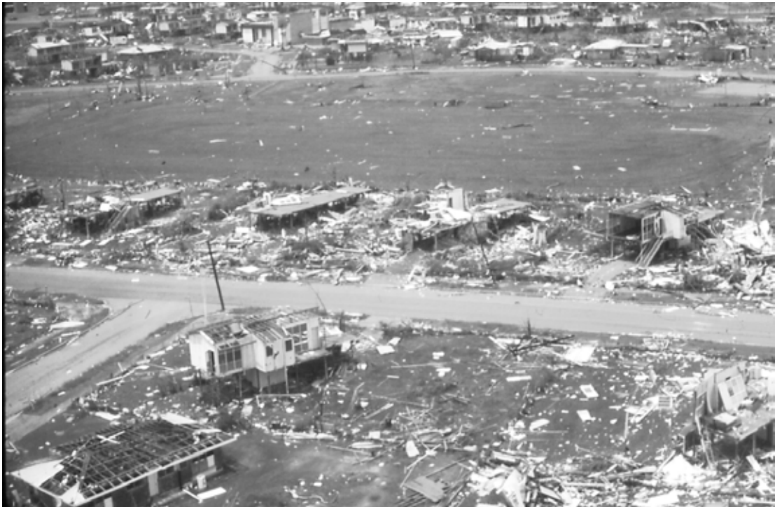
Fig 4.7 - Housing Damage from the Air
