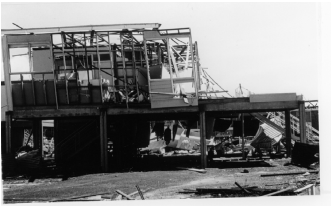
Fig. 5.8 - Typical half demolished house
