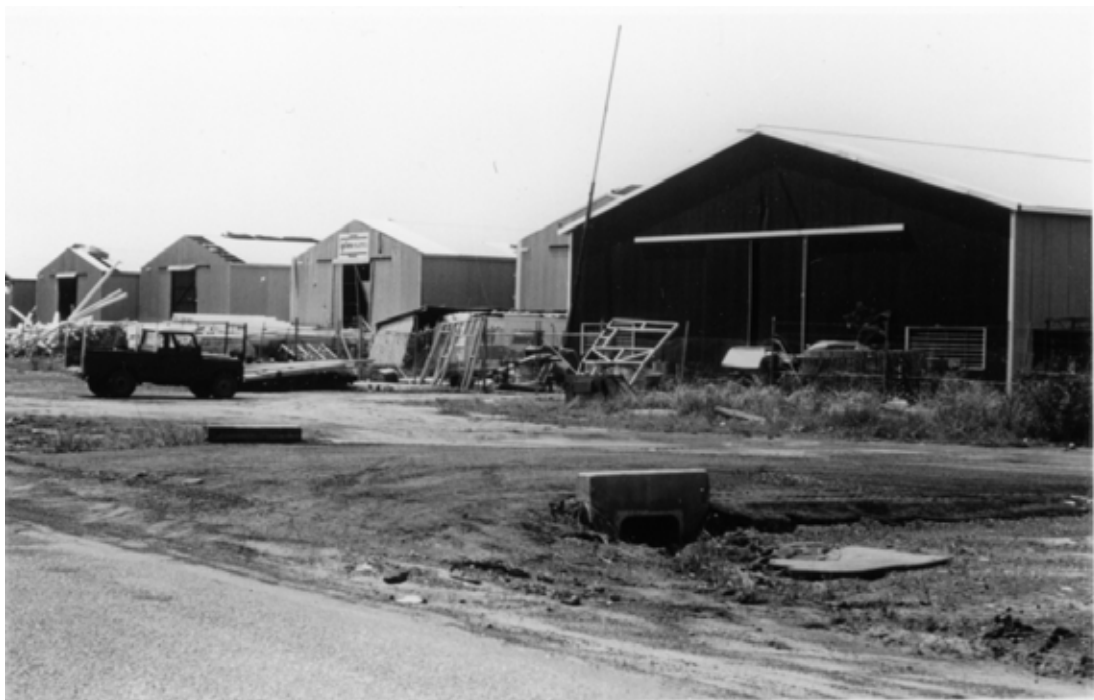
Fig. 5.6 - Typical industrial buildings
