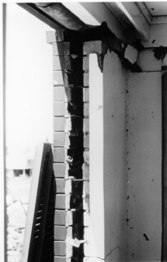
Fig. 5.15 - Lifting of bond beam
