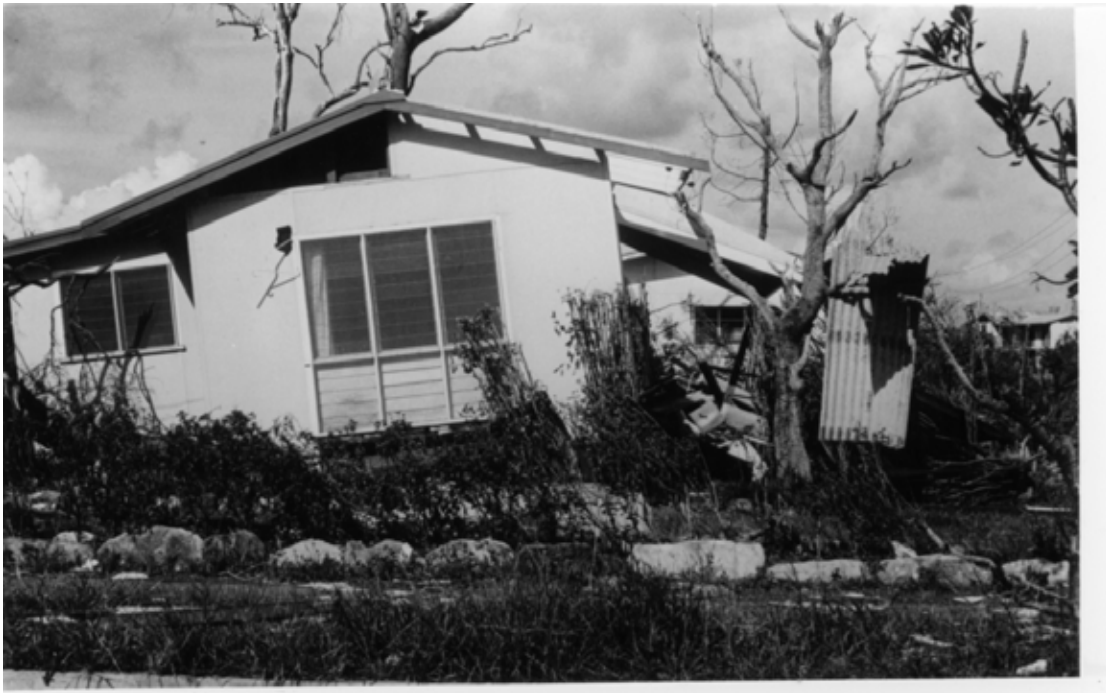
Fig. 5.9 - Pier collapse
