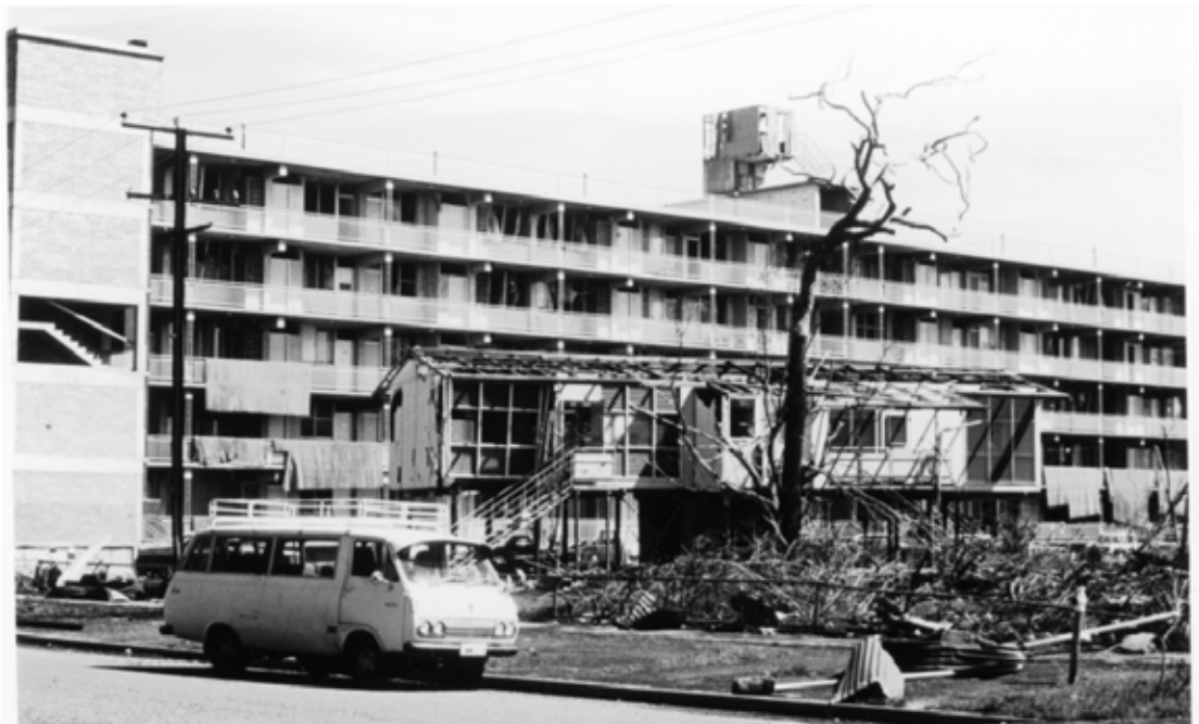
Fig 5.19 – Flats which performed well
