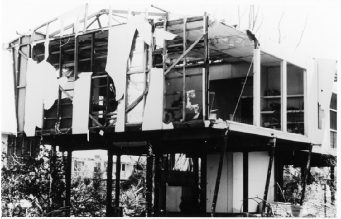
Fig. 5.22 - Battered wall cladding
