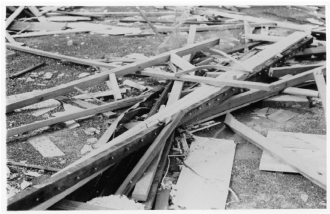
Fig. 5.3 - Screw fastenings remaining in purlin
