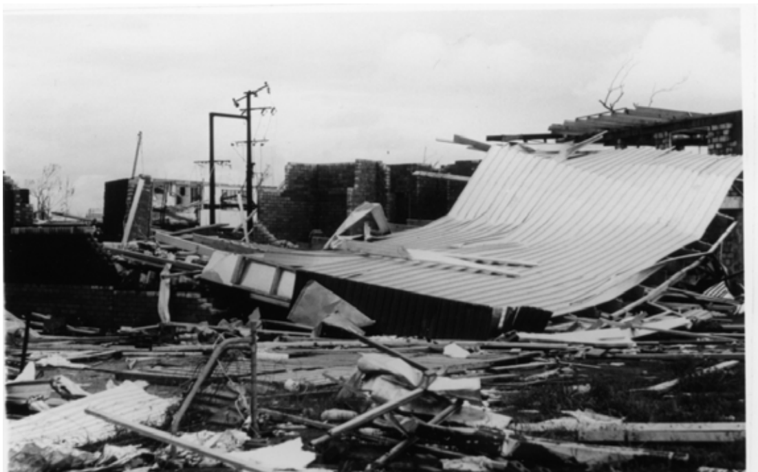
Fig. 5.4 - Failure of roof structure as a whole
