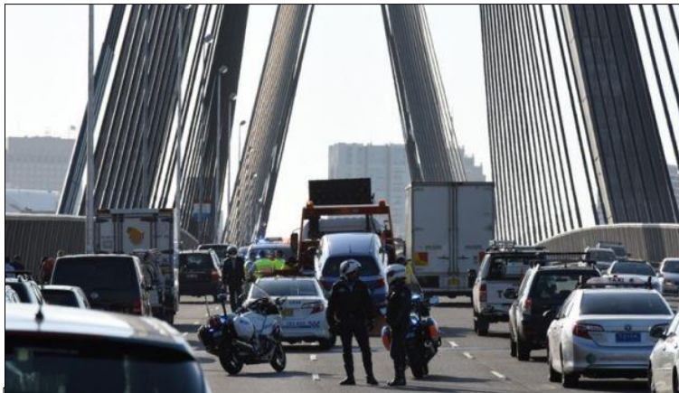
Cars and other vehicles traveling on the ANZAC Bridge.
