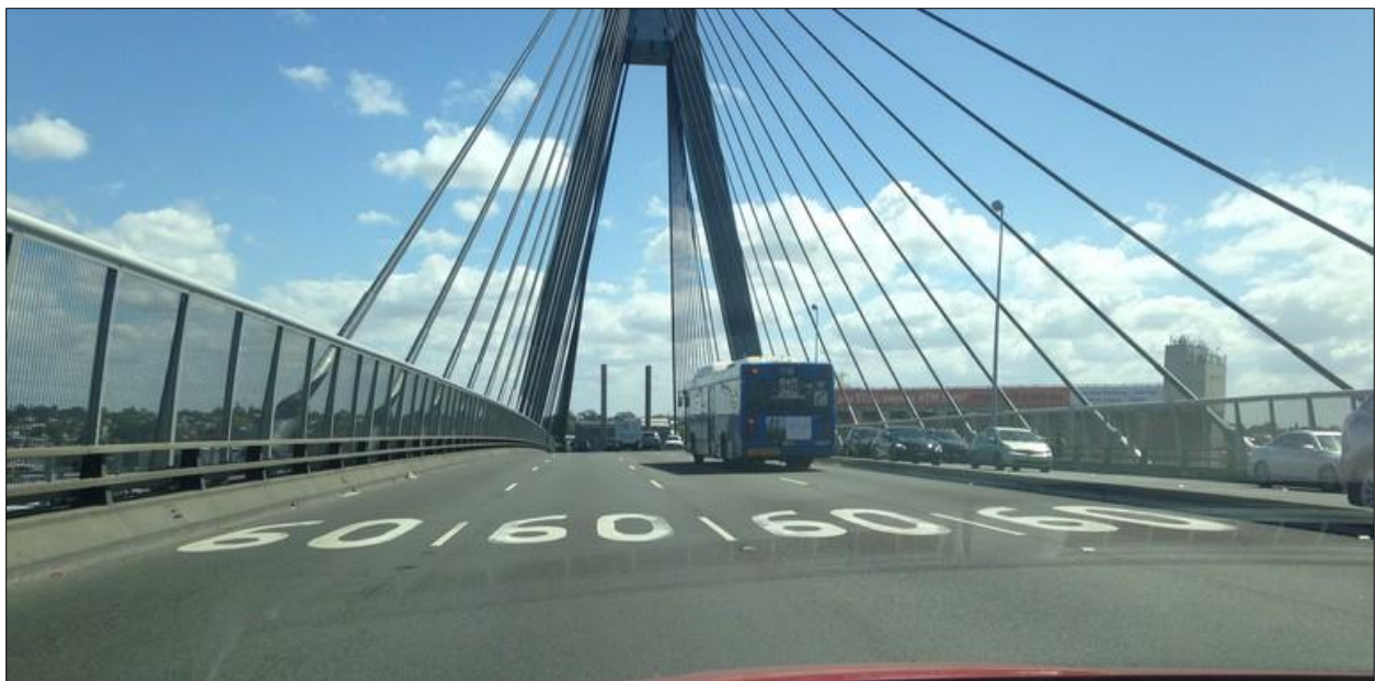
60 Speed Limit signs painted on the ANZAC Bridge road.
