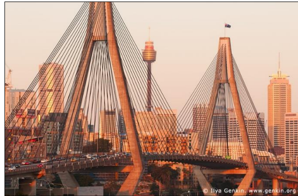
Two delta shaped towers of the ANZAC Bridge.
