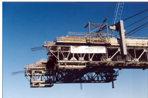
Formtraveller on the western deck
