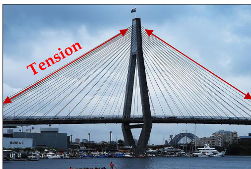
Stress in Stay Cables of the ANZAC Bridge.
